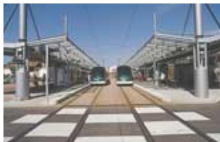
France - Applications Routières Tramway de Strasbourg.
