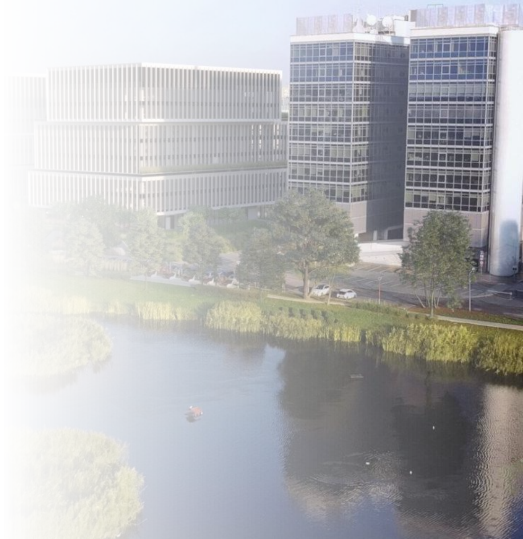
The Lakeside Project office complex in Warsaw, Poland, built using ECOPact with recycled construction demolition materials inside
