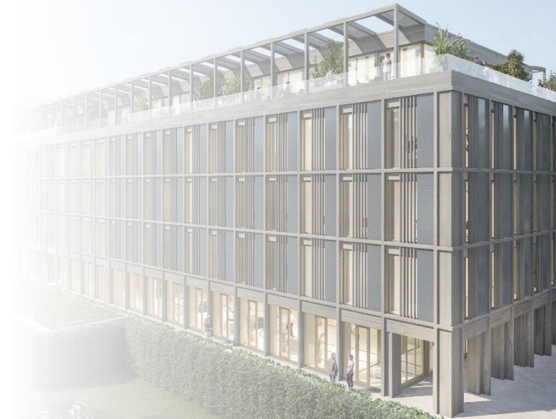
European Patent Office in Vienna, Austria built with ECOPact low-carbon concrete (with ECOCycle® inside) & Elevate ISOGARD™
