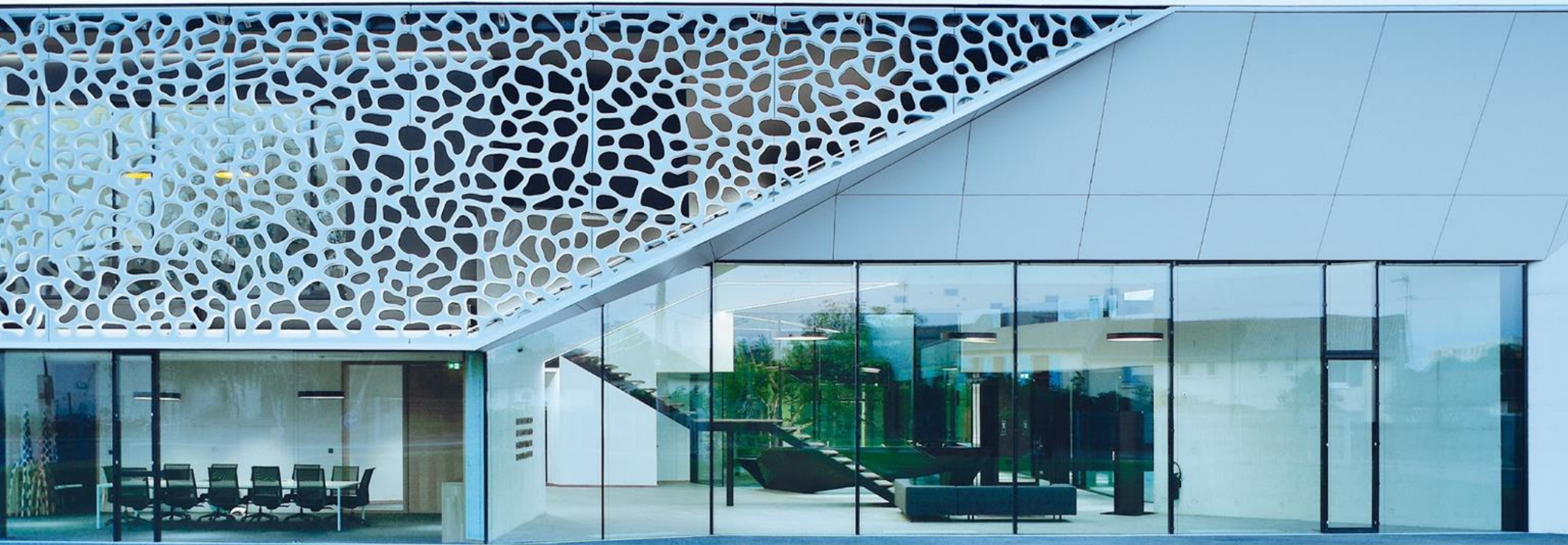
Cepovett head office in Gleizé, France. Built with Ductal inside.
