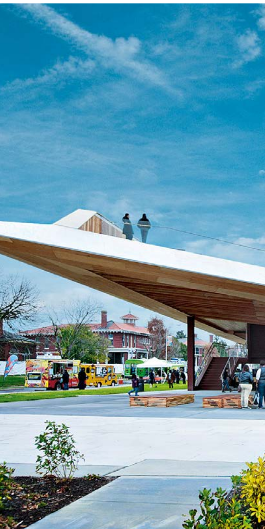
◀ Gateway in Washington D.C. built using Holcim ultra-high performance concrete.
