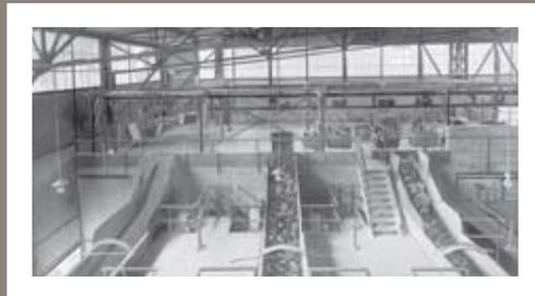
Limestone excavated in the quarry arrived at the plant via a cable car and was processed here.
